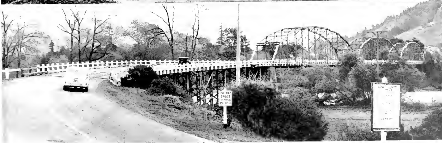
The massive structure shown above replaces unsafe Robinson Ferry Bridge across Eel River pictured below, posted for load limit
